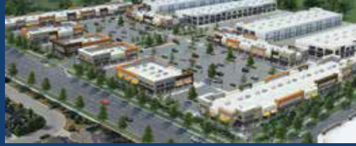
ERIN MILLS COMMERCIAL CENTRE PHASE II
